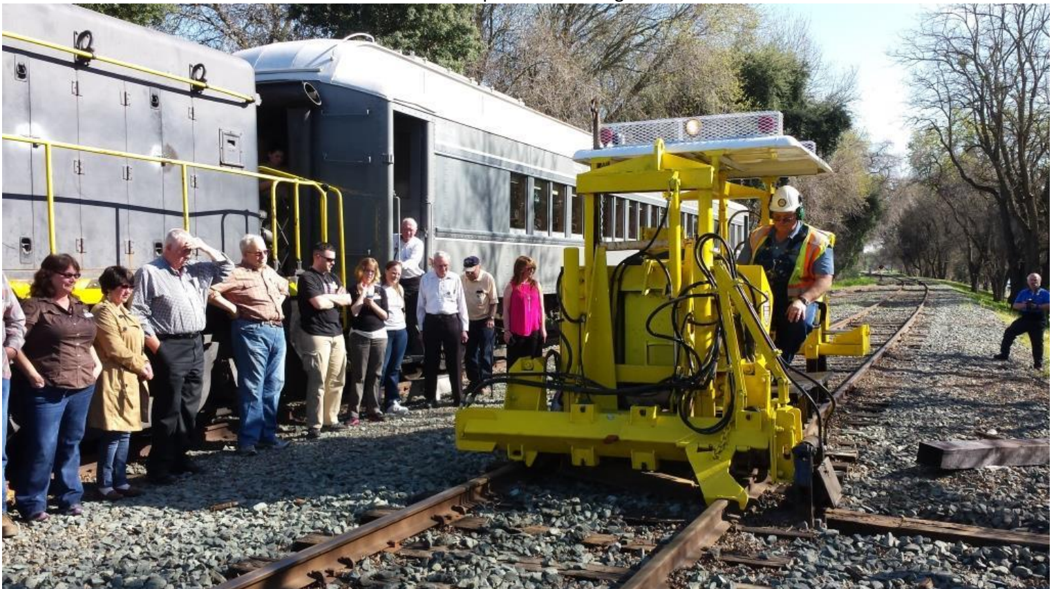
We've got a tie exchanger, scarifier, and tamper. Let's put on a show! Act 1: Chris pulls a tie with the 125
