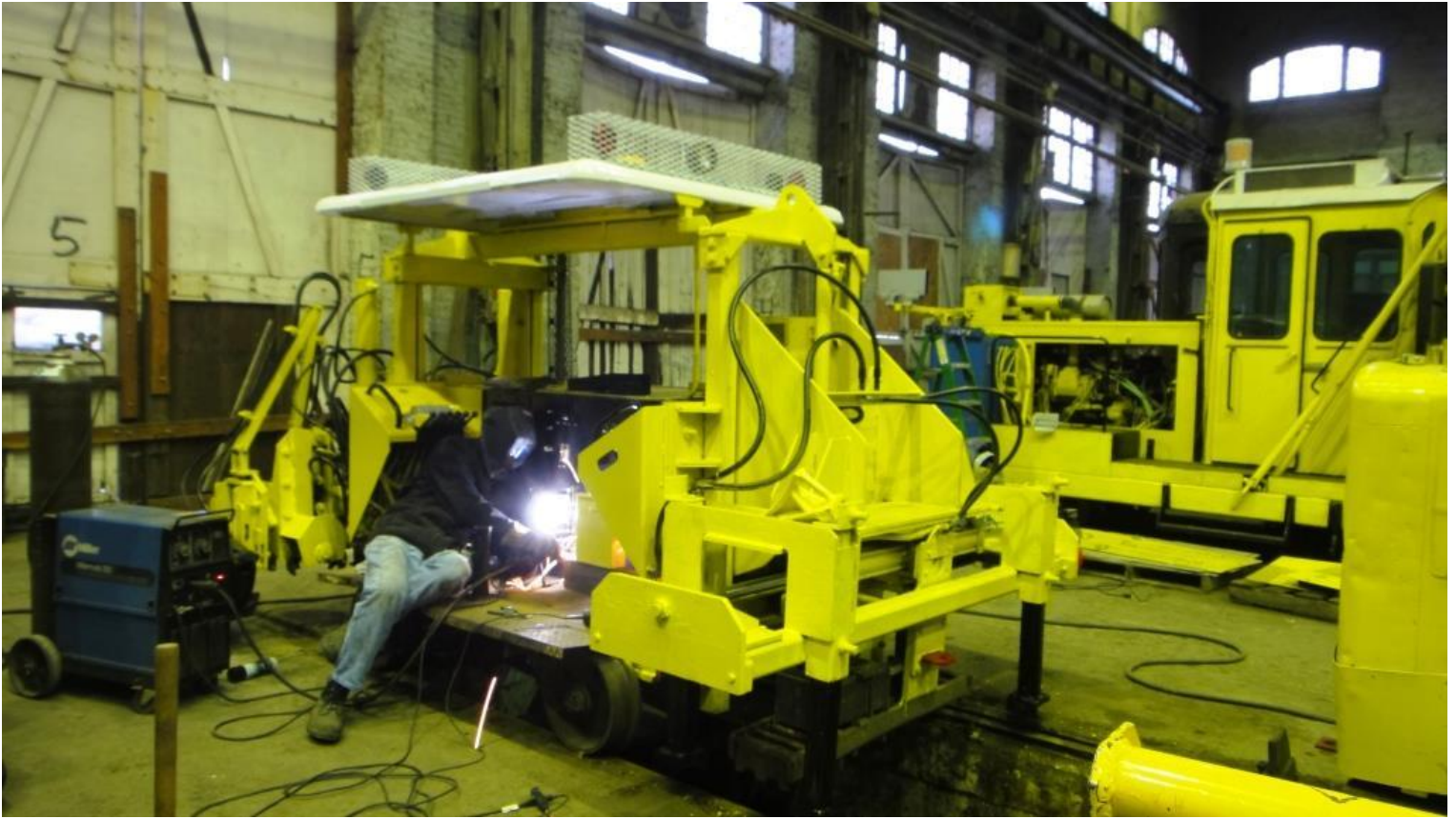
Alan welds a new secure lock-box on the Jackson 125 tie exchanger
