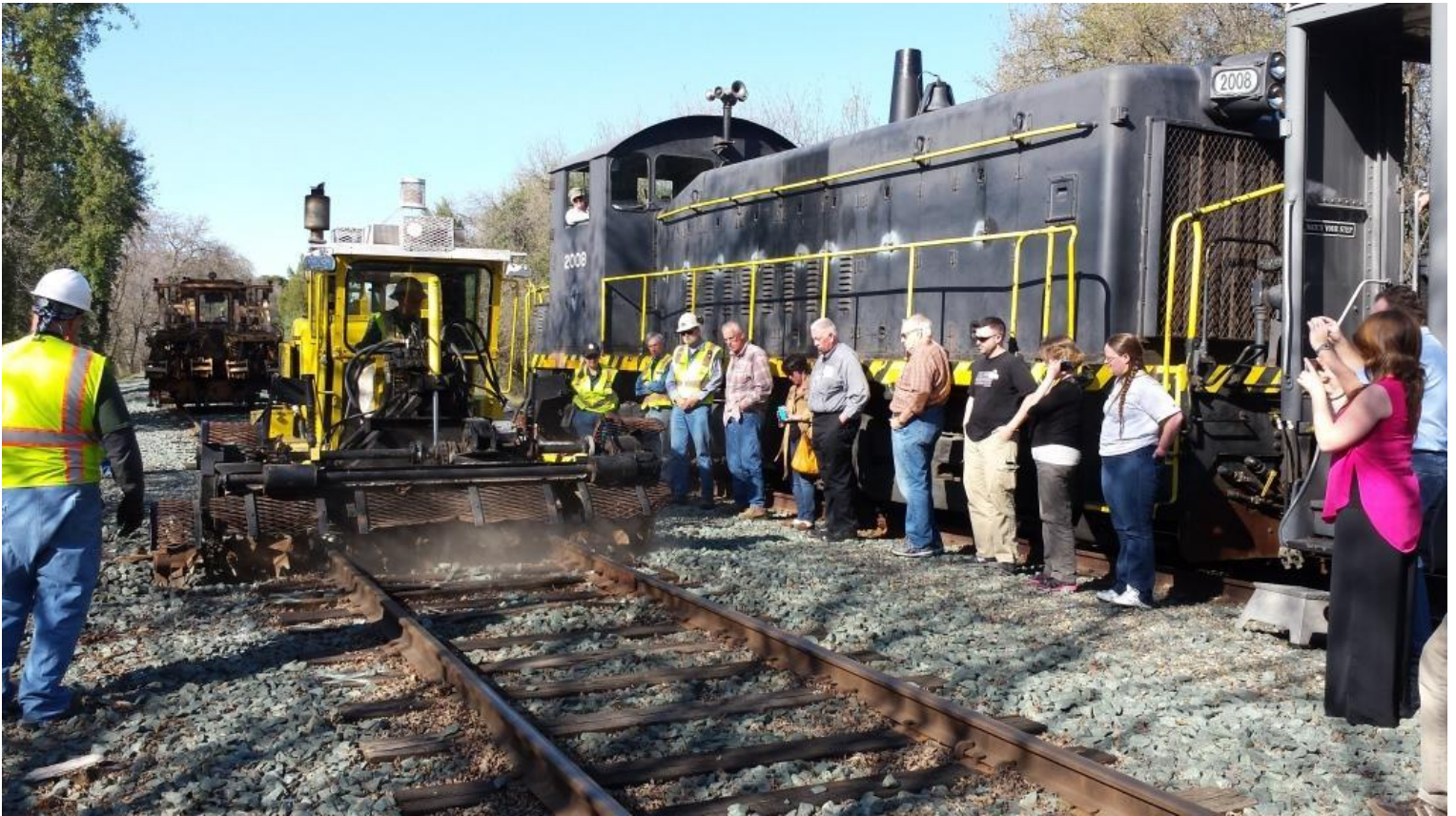
In the second act, Mike H. digs out the crib and inserts a new tie with the Scarifer/Inserter
