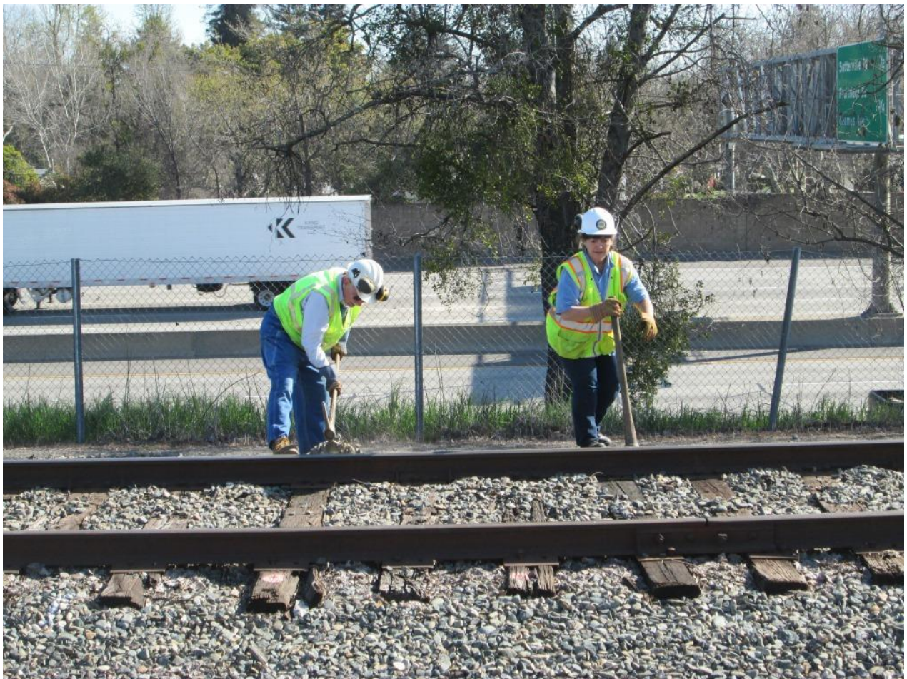
Clem and Pam dig out the ends of ties so that the Jackson 125 tie exchanger can get a good grip the ends
