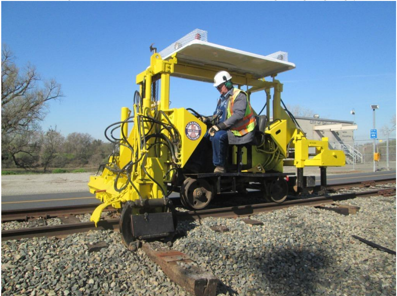
Chris at the controls has the 125 pulling ties like nobody's business!
