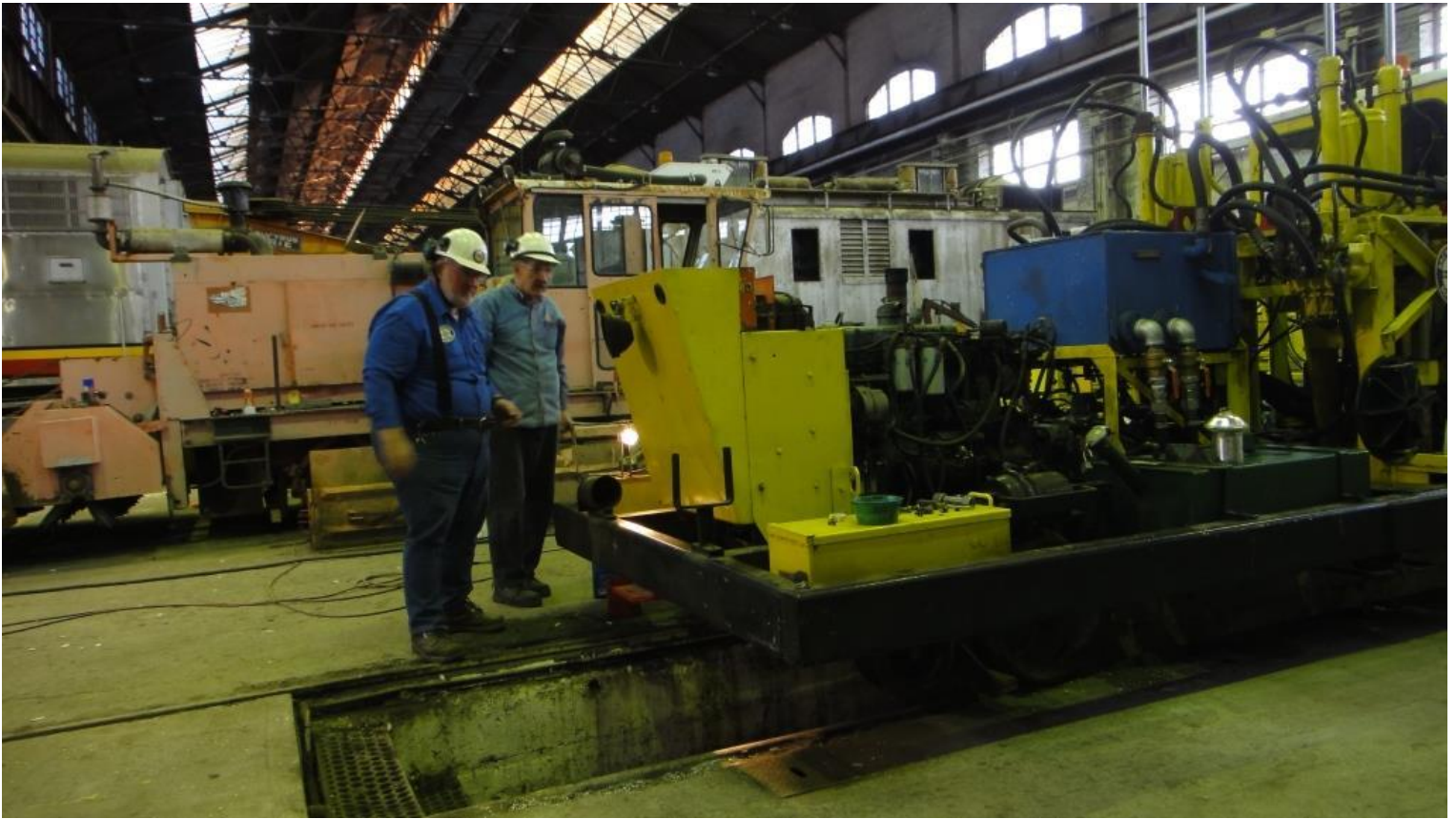
Frank and Fred reinstall the radiator shield on the tie shear
